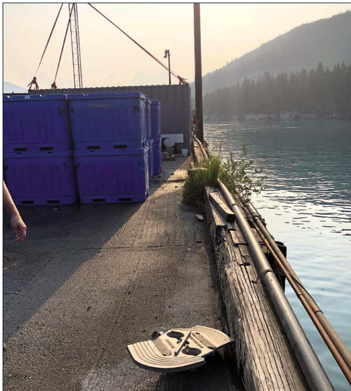
The portside hatch from the Alaganik, as found on the pier after the explosion. U.S. Coast Guard photo
